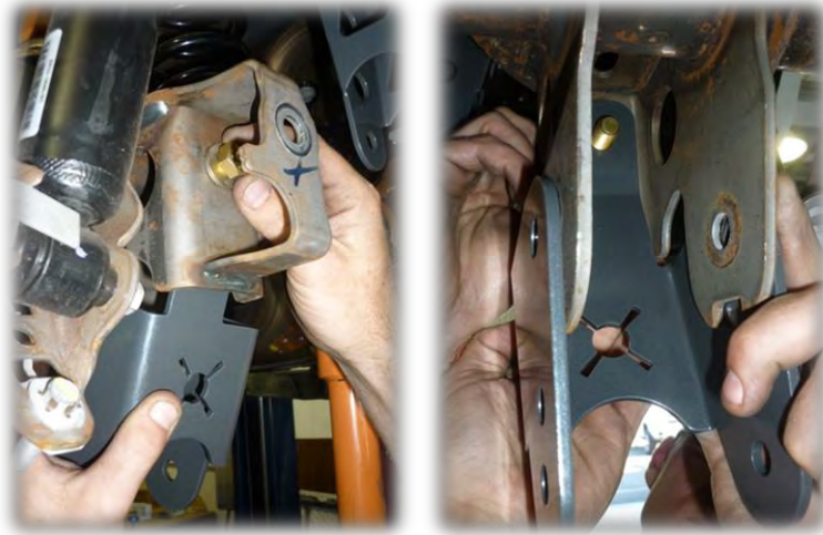
Figure 8: Driver Side Axle Bracket Upper Bolt Installations.
